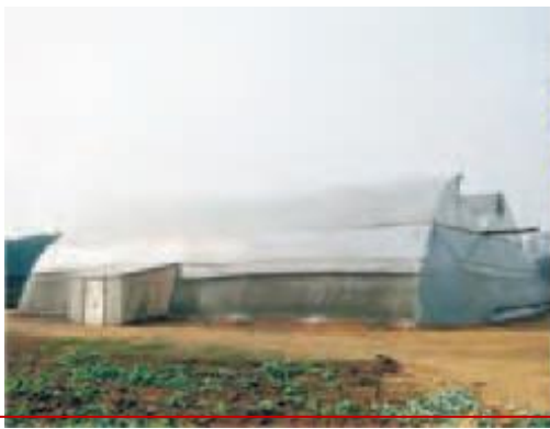
Naturally ventilated greenhouse for growing tomato and cucumber
